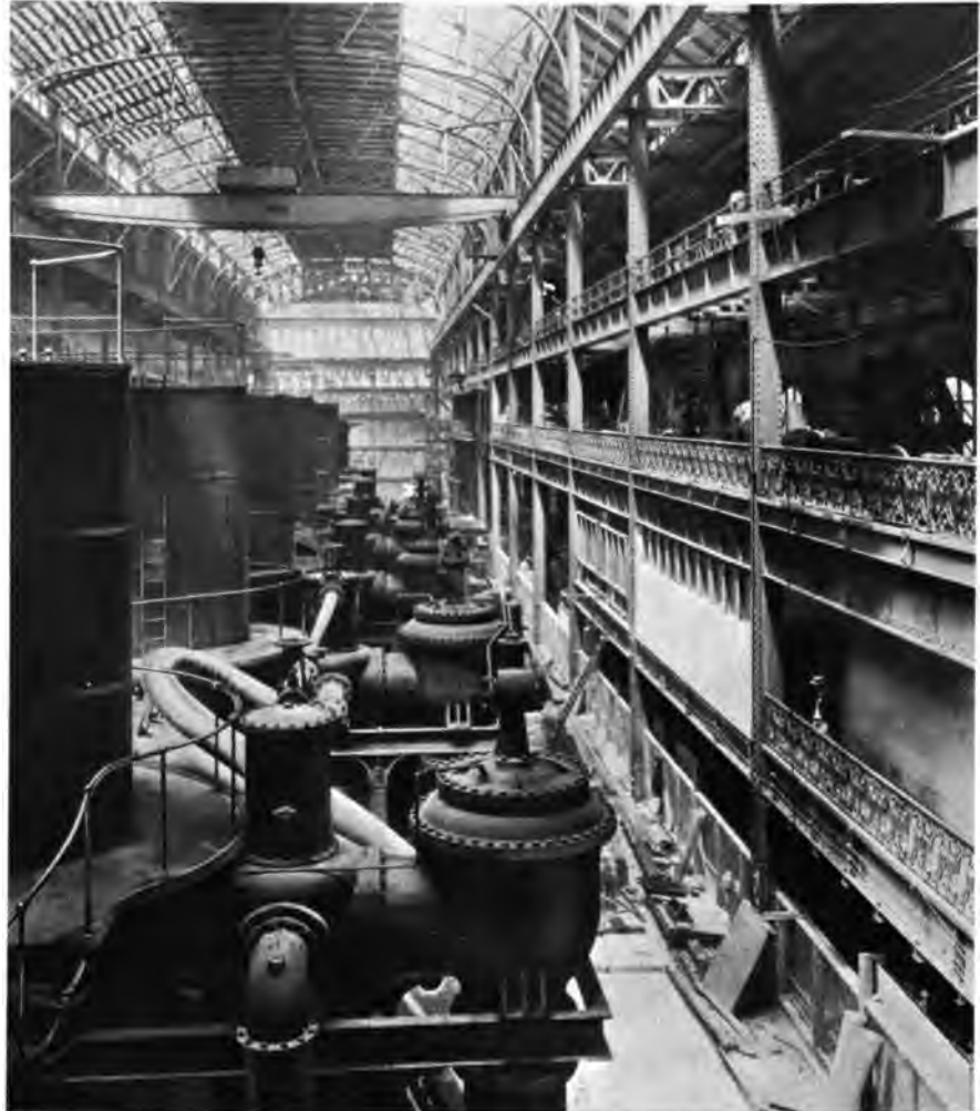
OPERATING ROOM SHOWING CONDENSERS — POWER HOUSE
